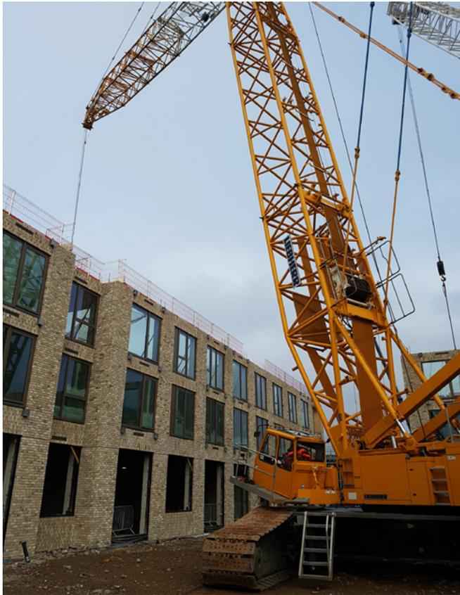
A 'total prefab construction' approach was adopted. This consisted of an integrated system for both the structure of the building (floor slabs and internal walls) as well as the external envelope and façade.
